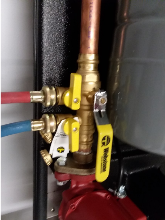
Valve Position to Run the System
