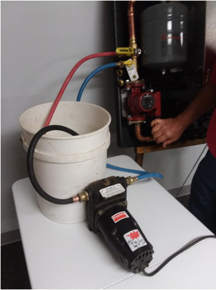
Filling the System using a Fluid Transfer Pump
