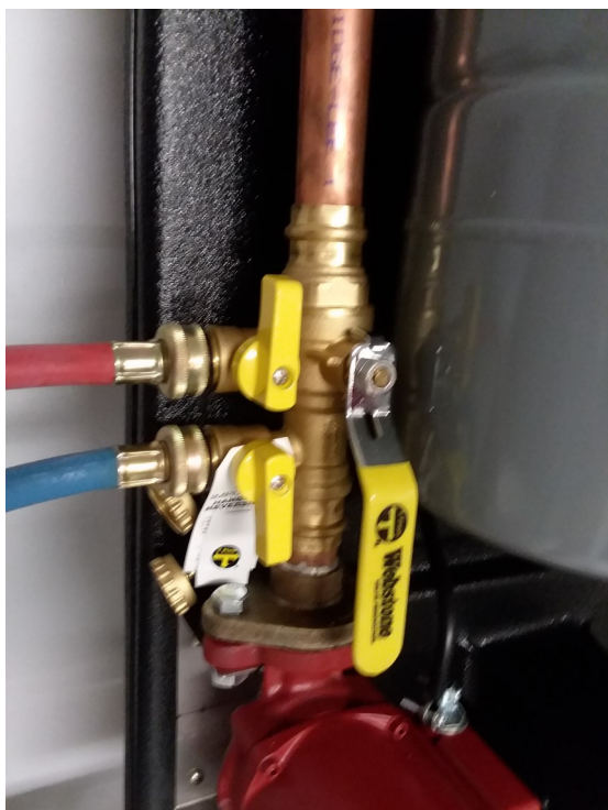
Valve Position to Run the System
