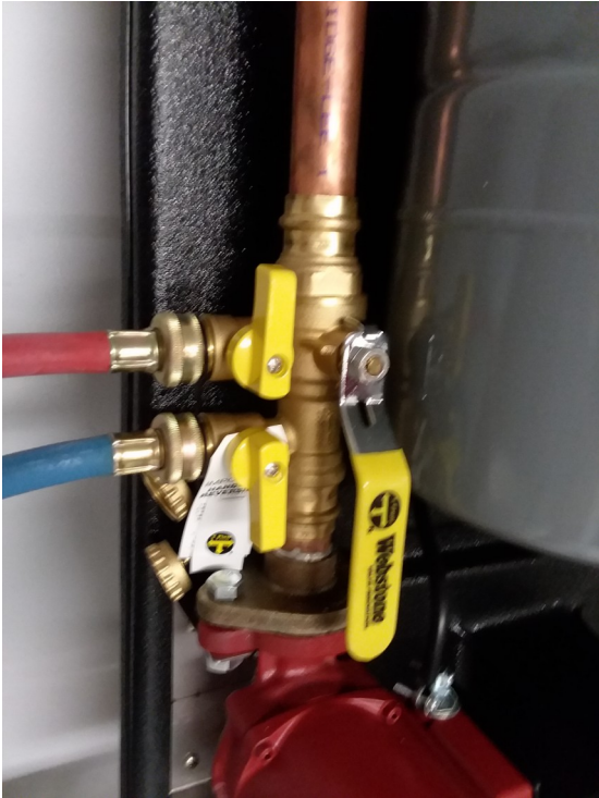
Valve position to run the system
