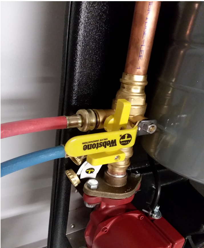
Valve position to pressurize the system
